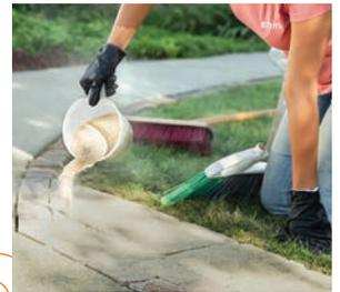
9 Lay down polymeric sand. Use push broom to push into seams and wet down with hose.
