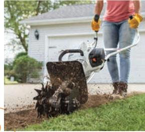
2 Once the grass is removed, use the MM 56 C-E YARD BOSS® to loosen up the dirt, making it possible to move and level ground 6" below the driveway.
