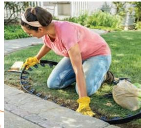
8 The outside pavers should be locked into space with an edge. You can do this by using a plastic paver edge with stakes.
