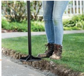
4 Add in a minimum of 4" of Class 2 base gravel. Use tamper to compact and level.
