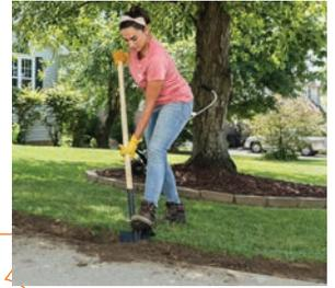
3 Use a shovel to roughly dig and level out. Over excavate so it's at least 6" wider than the paver design. Compact and level off the dirt.
