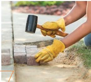
7 Use a rubber mallet to tap your pavers into the sand to level and make as snug of a fit as possible. Continue the process all the way to street.
