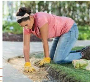
5 After the base gravel is even and level, add in around 1"-2" of paver sand (not playground sand as it doesn't compact as well as a paver sand layer). Use tamper to compact and level the sand.
